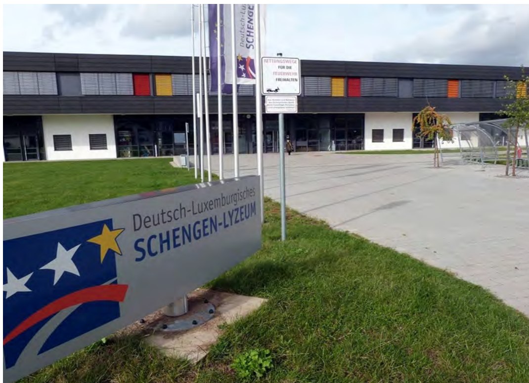
The entrance to the school building
