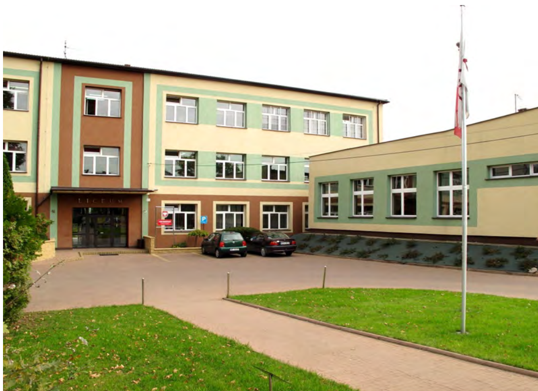
The entrance to the school building
